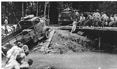
Fig. 2 Pulling vehicles across a waterway near Penang.
